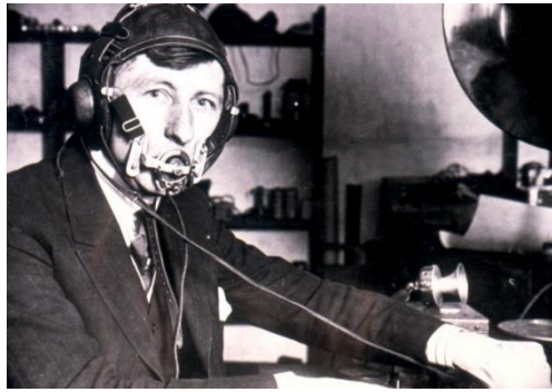
02 Peter Laurits Jensen demonstrating the noise neutralizing microphone and headset used by the US Navy during World War I.
